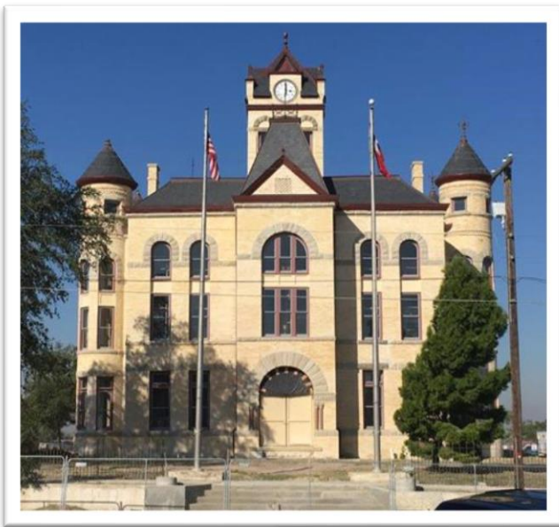
Figure 3-2: Karnes County Courthouse (after restoration)
